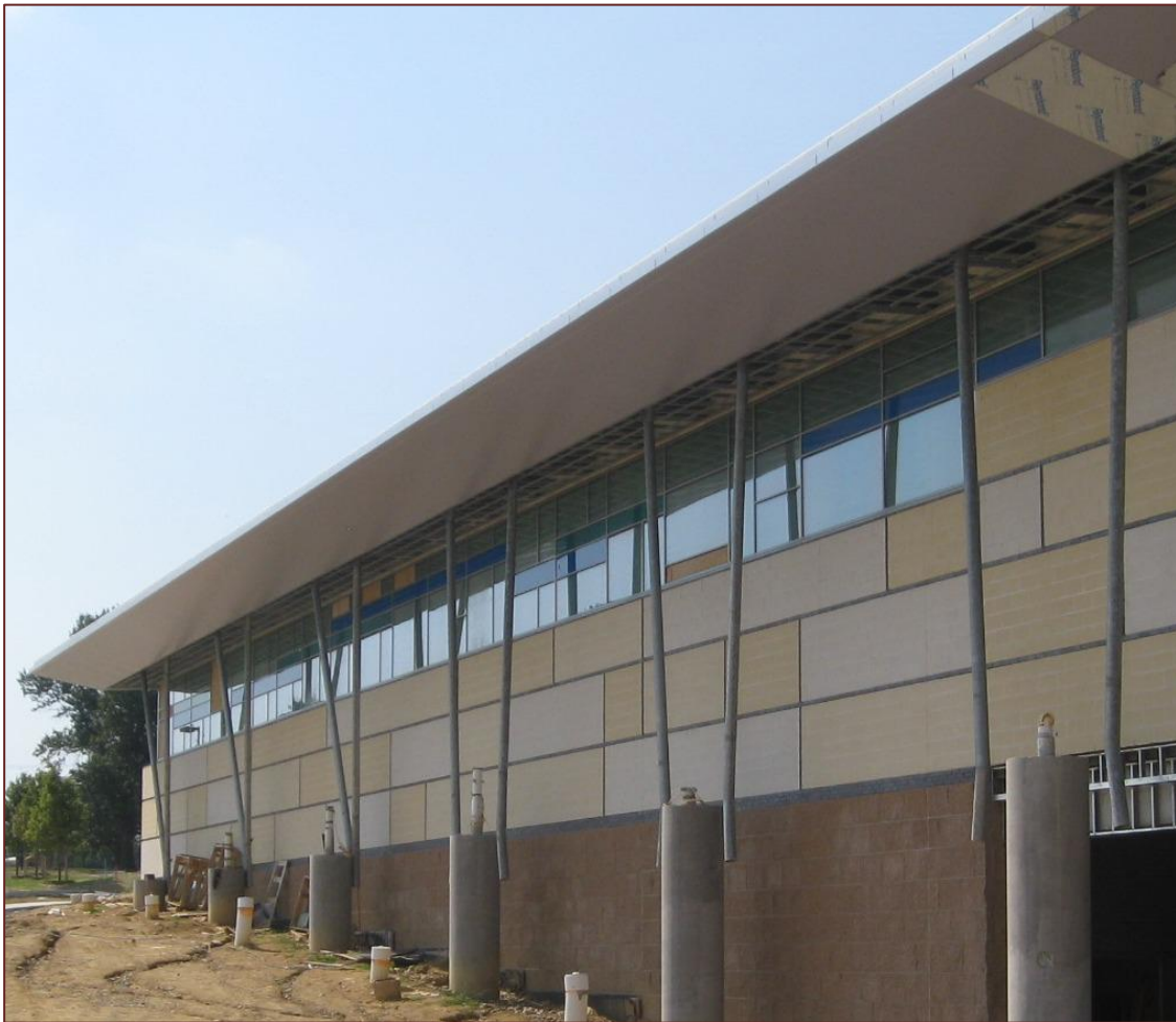
Figure 1: Drainage pipes along the south side of the basketball arena. The pipes create an architectural feature and functions as a roof rainwater collector.
